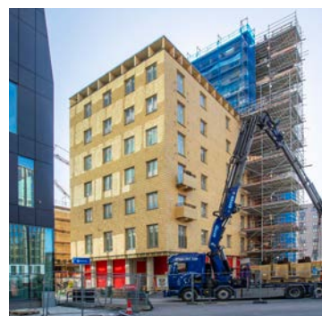
Stockholm's first large-scale apartment block in mass timber under construction. Hagastaden.
